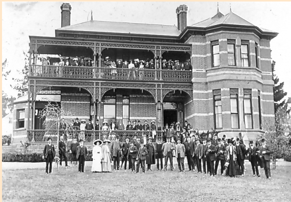
School of Forestry, Creswick. Courtesy of DSE.
